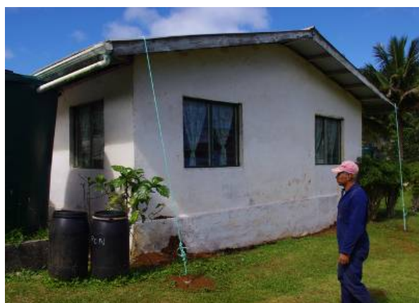
Figure 3: A house with the roof anchoring system.
